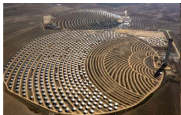
Picture of PS 20 still under construction (©Abengoa)
